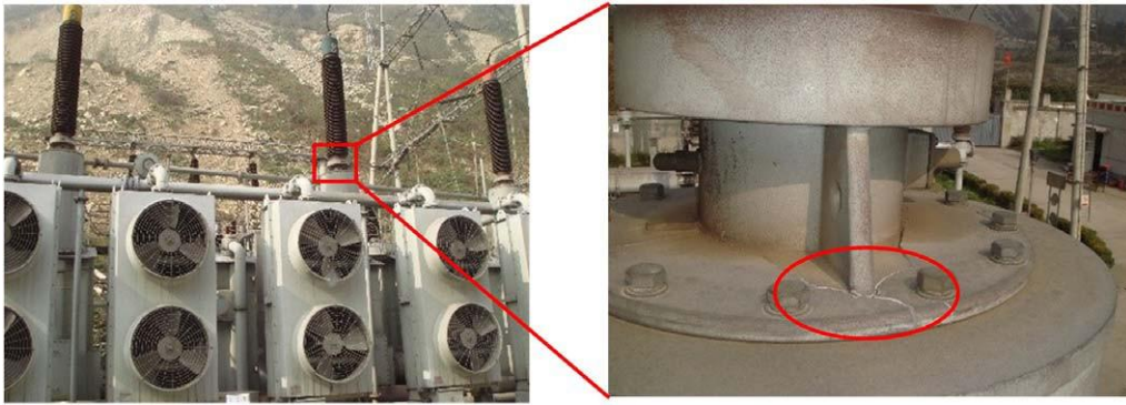
Figure 1. Failure of the metal flange of a 220-kV transformer bushing in the Wenchuan earthquake.
